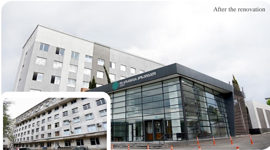
Before the renovation
